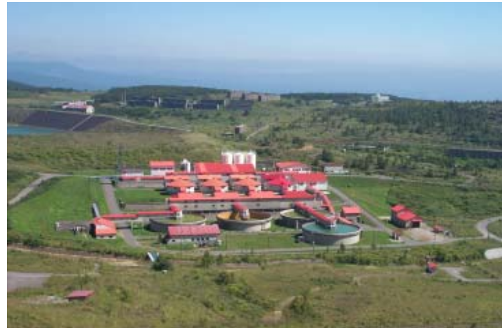
The Matsuo Neutralization Plant
