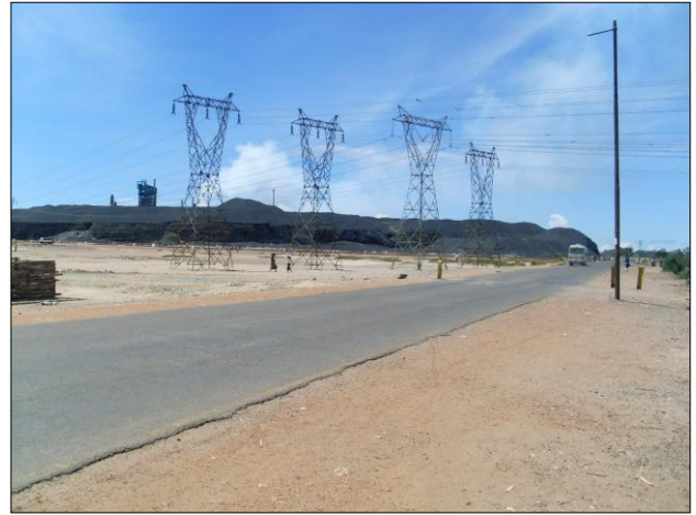
The area of slag heaps in Kankoyo to the west to the smelter, Mufulira, Zambia
